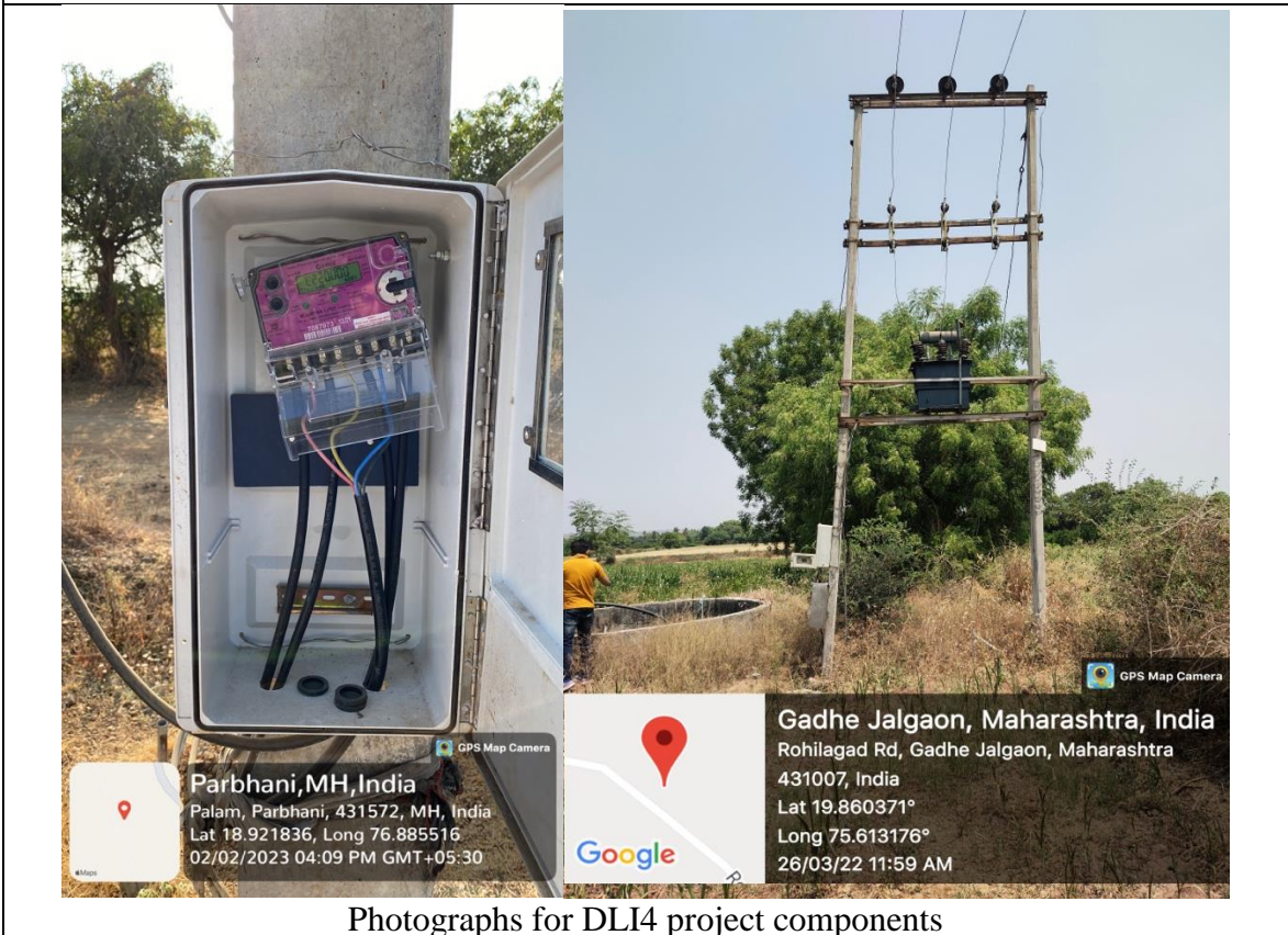
Transformer installed at new substation
