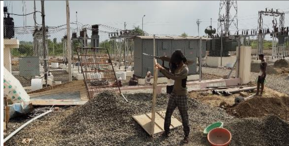
General construction practises at substations
