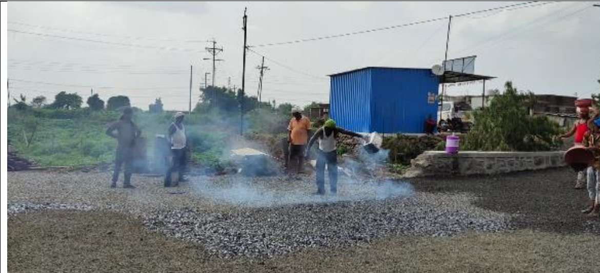
Bituminous Road construction within substation
