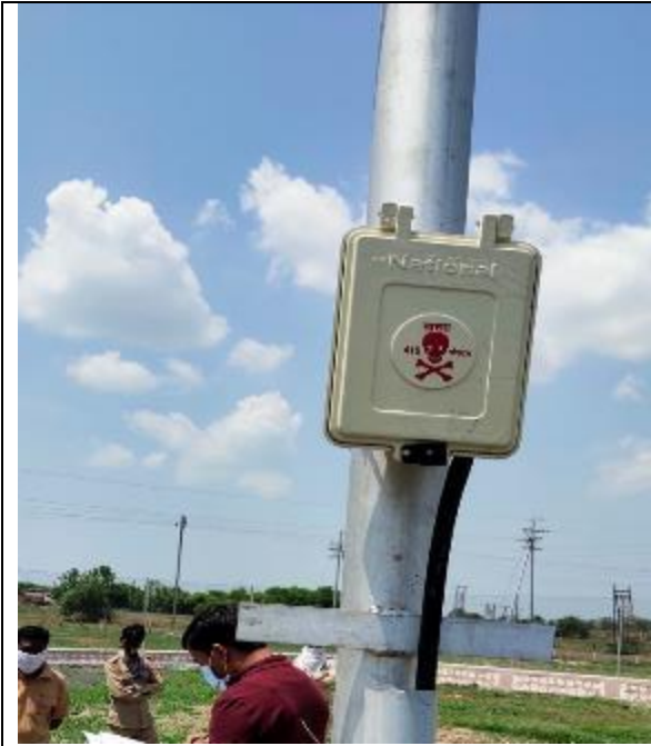
Danger board on poles
